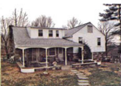
PENDING DEMOLITION. This 1959 Bryn Mawr, Pa. split-level was the first on its block to go.
